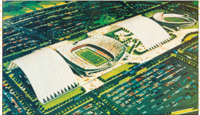
Original plans for the Truman Sports Complex called for a rolling roof which could cover Arrowhead or its baseball counterpart, Kauffman Stadium - a revolutionary concept at the time.
